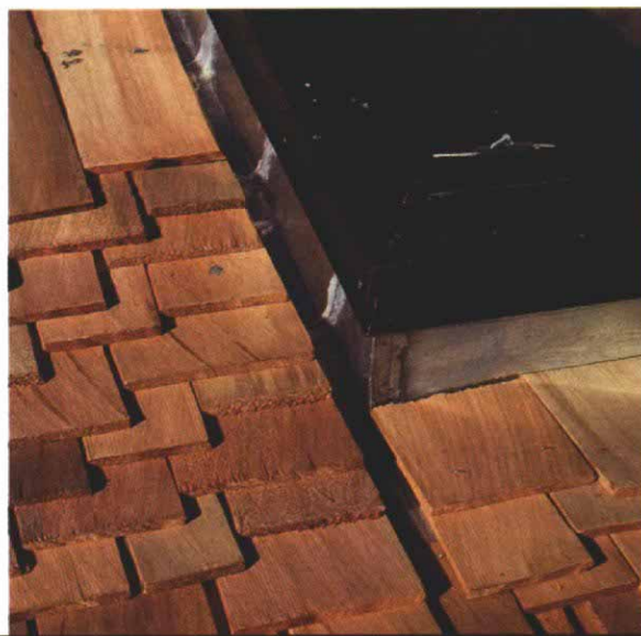
As with hips, shingles are installed over valleys in continuous courses, creating a smooth transition between adjacent roof sections. Valley shingles are fanned out so that the shingles touch only at their butt ends. Shingles are affixed with the aid of pneumatic staplers.
