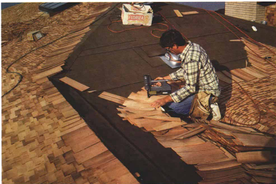
As with hips, shingles are installed over valleys in continuous courses, creating a smooth transition between adjacent roof sections. Valley shingles are fanned out so that the shingles touch only at their butt ends. Shingles are affixed with the aid of pneumatic staplers.
