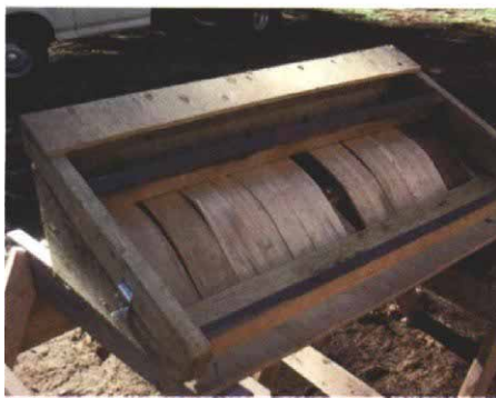
Shingles for radiused eaves are steamed and bent to the proper curvature before installation. The author's steamer consists of a truck utility box modified to fit over a 55-gal. drum of boiling water (top photo). Once shingles are saturated with moisture and become pliable, they're transferred to the bending jig (middle photo). When the jig's lid is closed, a pressure bar in the lid forces the shingles to bend over a platen to the proper radius (bottom photo). Typically, about 10% of the shingles break while bending.
