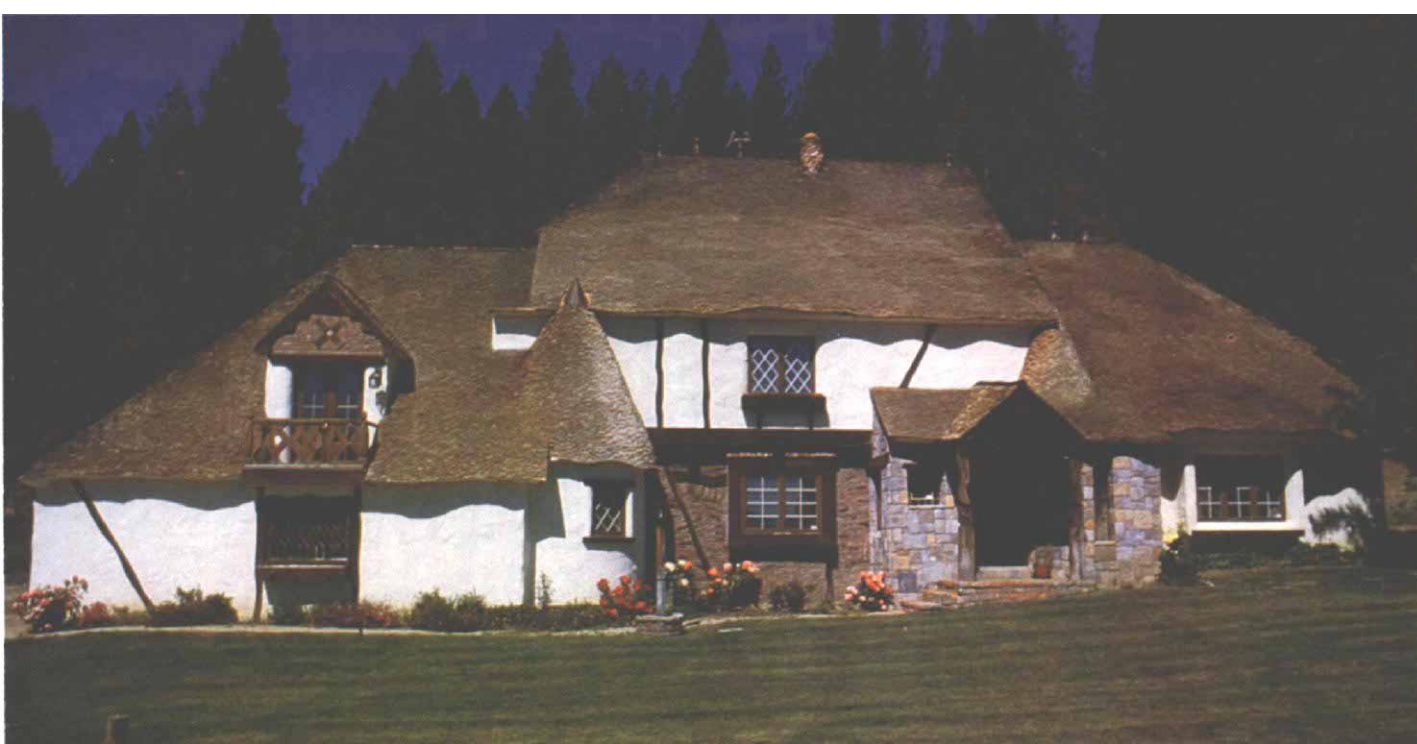
Instead of radiused rakes and eaves, some roofs terminate at square roof edges. As shown in the photo above, wave-coursing was used for the starter courses to create an authentic droopy appearance.
